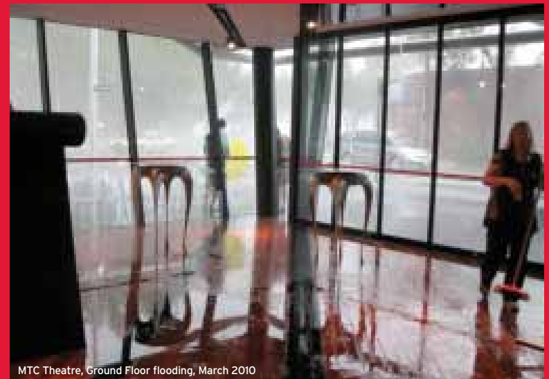
MTC Theatre, Ground Floor flooding, March 2010
